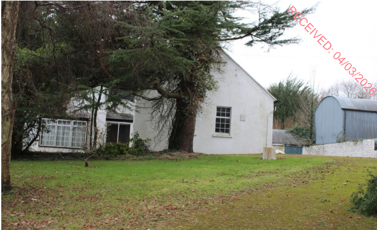
Fig. 15: 7: Farm house and yard on west side of development
