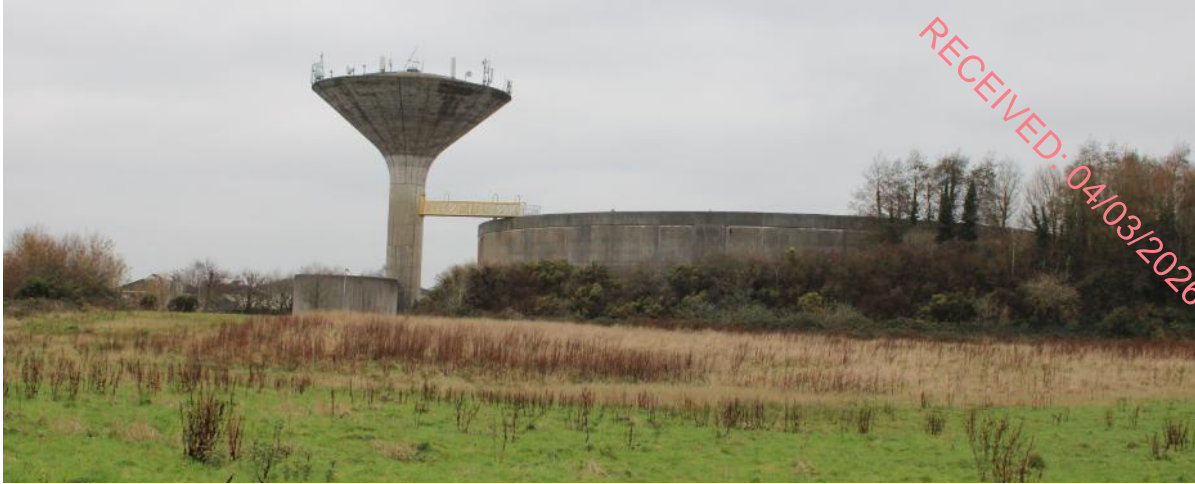
Fig. 15: 9: Newcastle Reservoir (Looking North)
